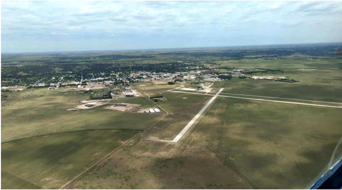
Valentine airport in Nebraska, with its two runways. Runway 3 is in the foreground.
